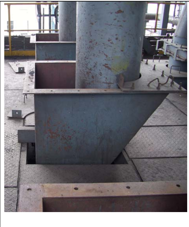
Photo 12: The fuel feeding on the left side is what is in this plant. The weight of the coal acts on the feeder. It makes cakes of coal. The one on the right is what is in another plant. The coal slides through by virtue of the hydrostatic head of coal. The lump formation will be avoided.
